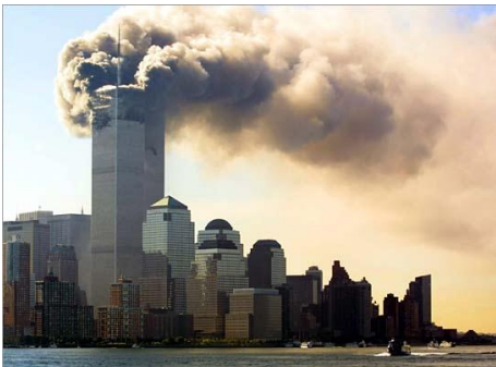
Fig.2.9. Tower of the WTC continue to resist to the effects of fire after the impact of the plane and the explosion of fuel
