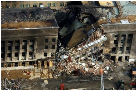
Fig.2.15. The progressive collapse of the outer rings in the Pentagon building (09.11.2003)
