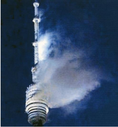
Fig.2.3. The fire on the Ostankino TV tower
