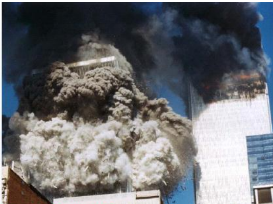
Fig.2.10. Beginning of the progressive collapse of the WTC-2 (South tower) after 56 minutes of aircraft attack
