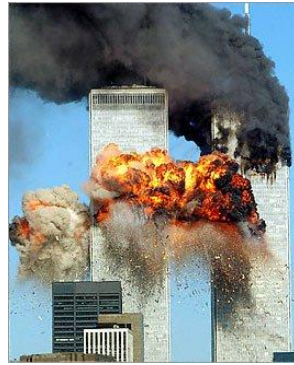
Fig.2.8. The explosion of the fuel in the zone collision of aircraft with the building of the WTC-2 during the terrorist attacks of September 11, 2001
