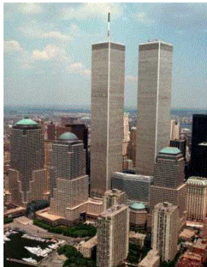
Fig.2.6. General view of the WTC towers, NY
